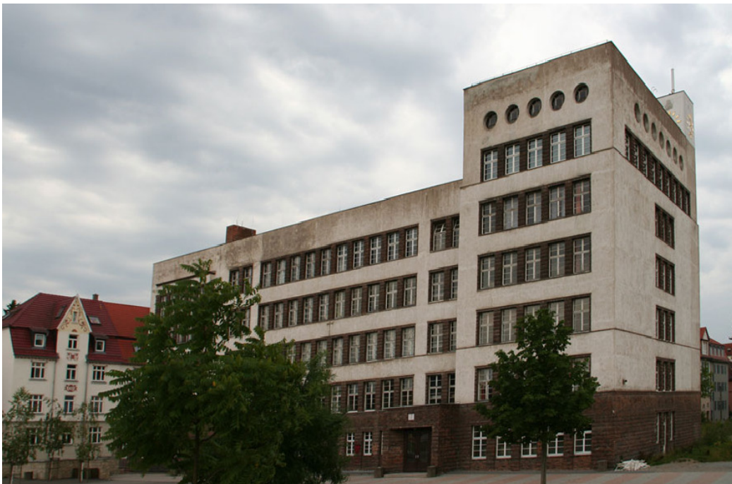
Figure 1. Friedrich Schiller Gymnasium in Weimar 2
