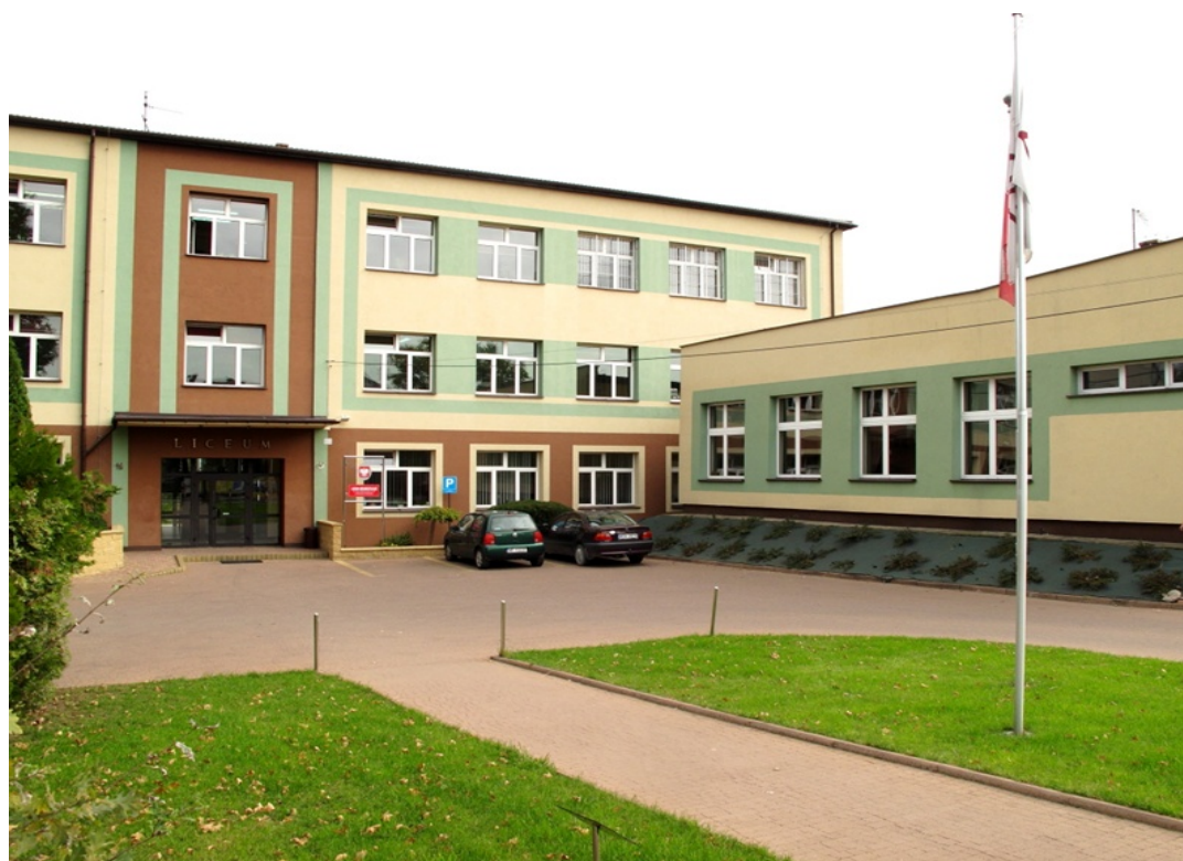
The entrance to the school building
